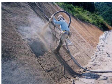
Shotcreting for Slope Stabilization
